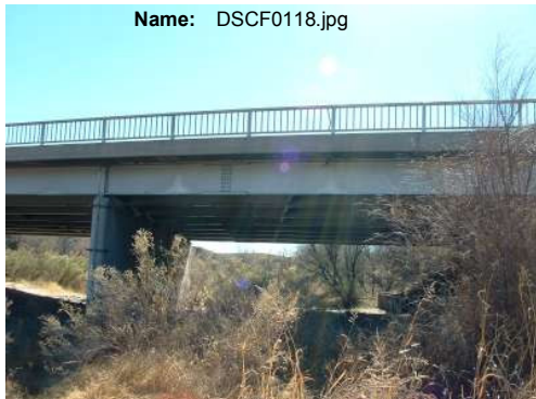
Azimuth: 158 Zoom: 1x Notes: I-10 bridge for Cienega Creek.
