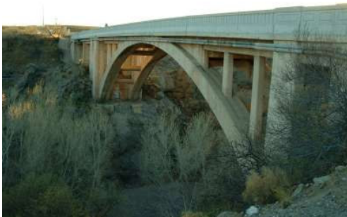
Azimuth: 210 Zoom: 1x Notes: Cienega Creek Marsh Rd./Railroad bridge.
