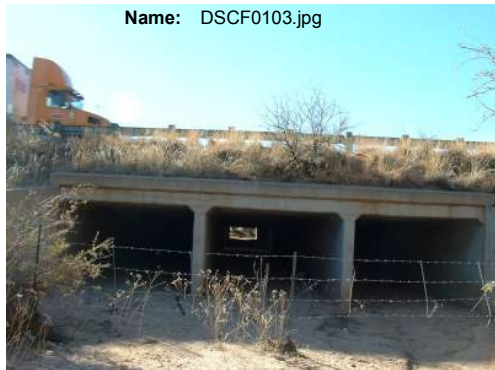
Azimuth: 182 Zoom: 1x Notes: Culvert under Cadillac Wash
