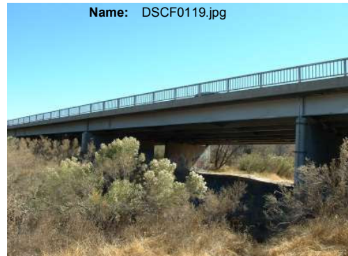
Azimuth: 132 Zoom: 1x Notes: I-10 bridge for Cienega Creek.
