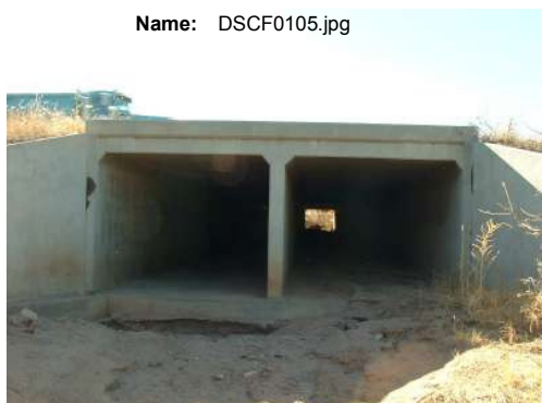
Azimuth: 176 Zoom: 1x Notes: Photo taken from I-10 culvert
