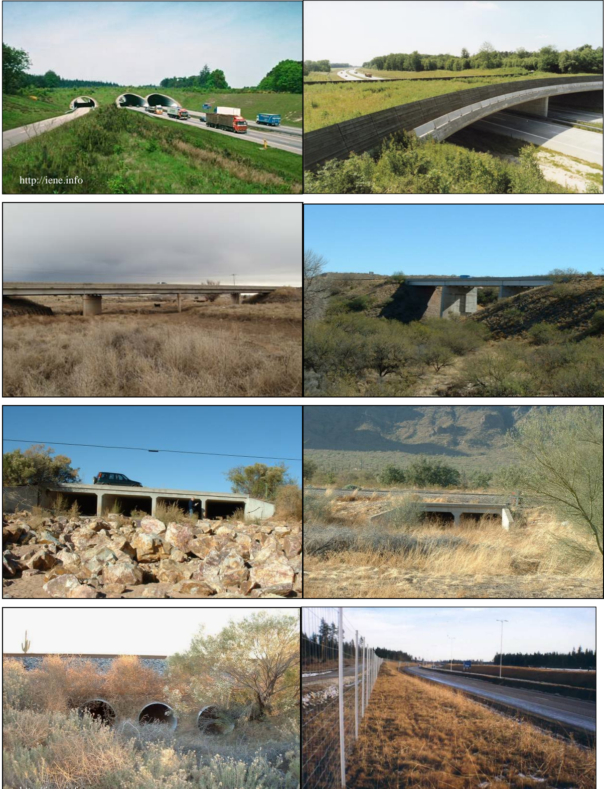
Figure 8: Potential road mitigations (from top to bottom) include: highway overpasses, bridges, culverts, and drainage pipes. Fencing (lower right) should be used to guide animals into crossing structures.
