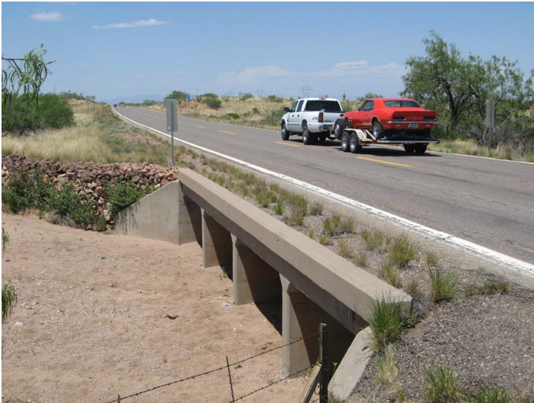
Figure 11: A 4-box culvert under US 191 at Milepost 96, Waypoint 64
