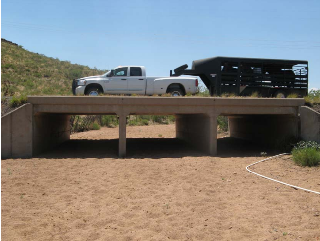
Figure 10: A 3-box culvert under US 191 at Milepost 95, Waypoint 63
