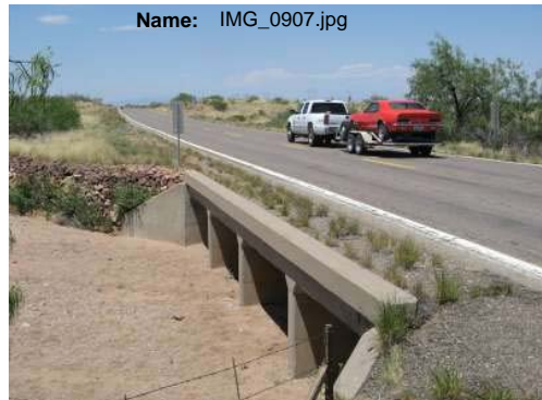
Notes: A 4-box culvert Zoom: 1
