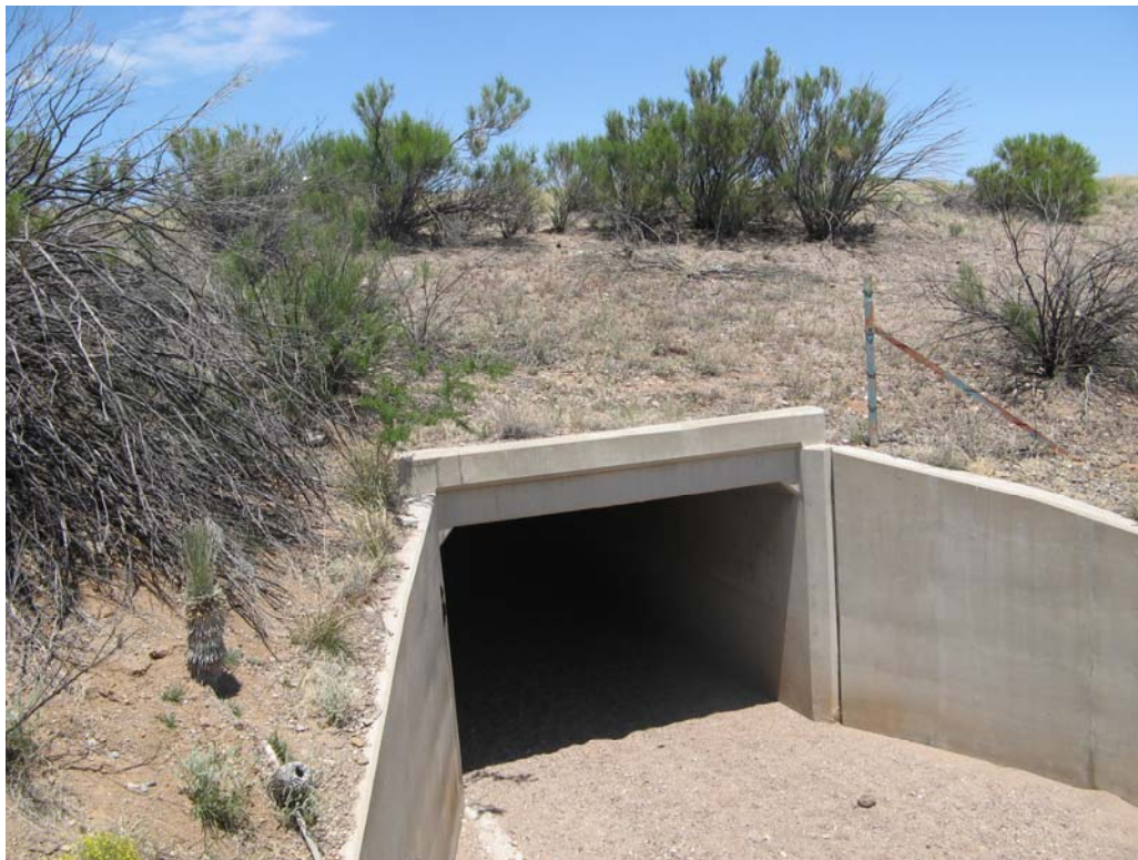
Figure 9: An 8x10' box culvert under I-10 at Milepost 351, Waypoint 59
