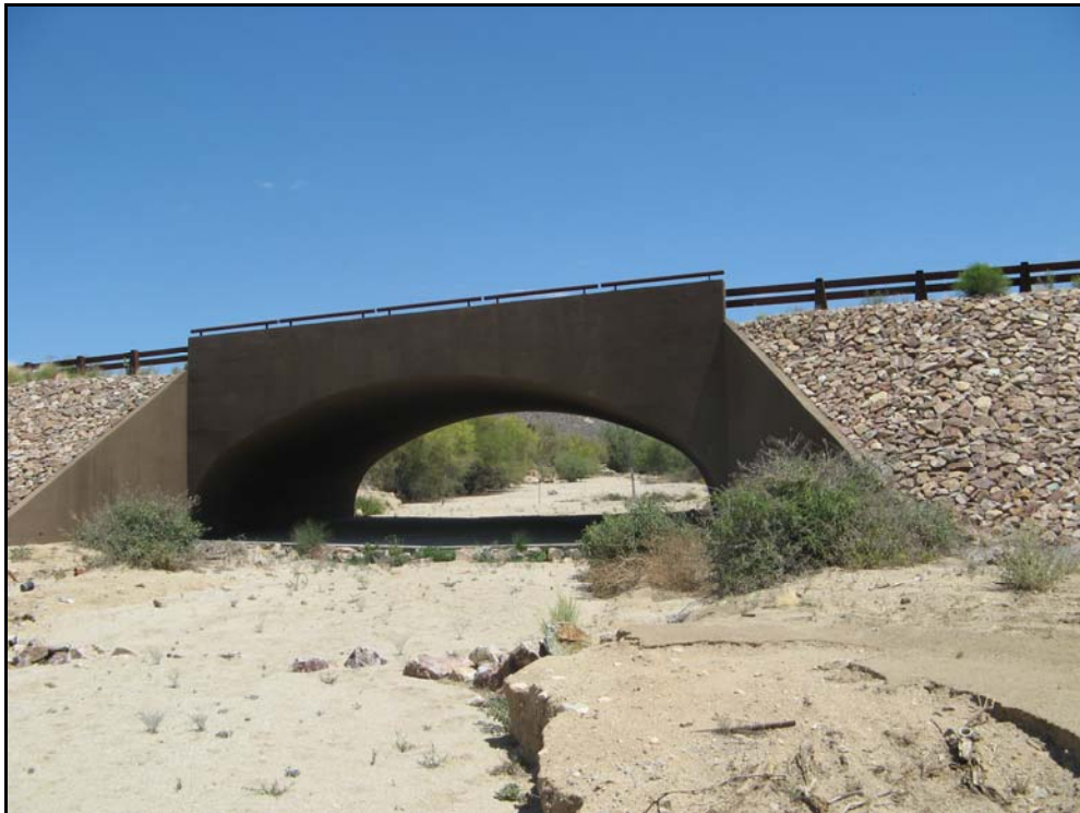
Figure 11: The bridge on Dove Mountain Road (Waypoint 19).
