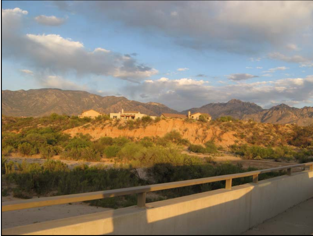
Figure 19: View to the northeast from the Rancho Vistoso bridge over Big Wash (Waypoint 11).
