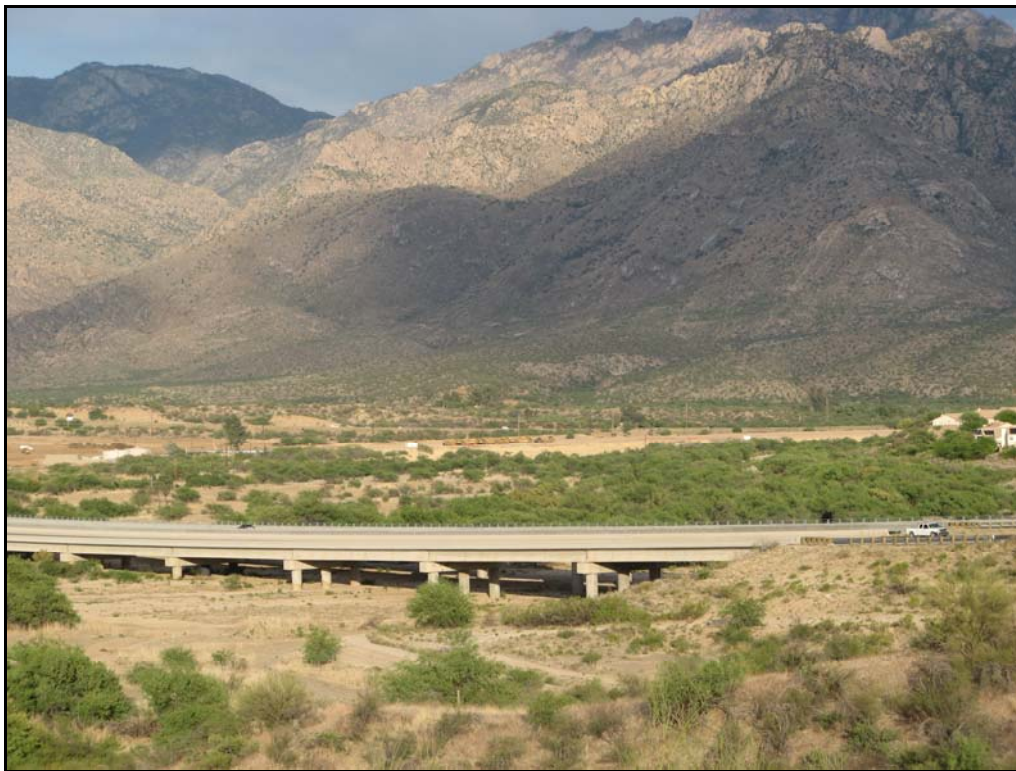
Figure 20: View downstream on Big Wash towards the Tangerine Road Bridge (foreground), SR-77 (linear feature in mid-field), and the Santa Catalina Mountains (on the horizon) Waypoint 9, looking southeast.
