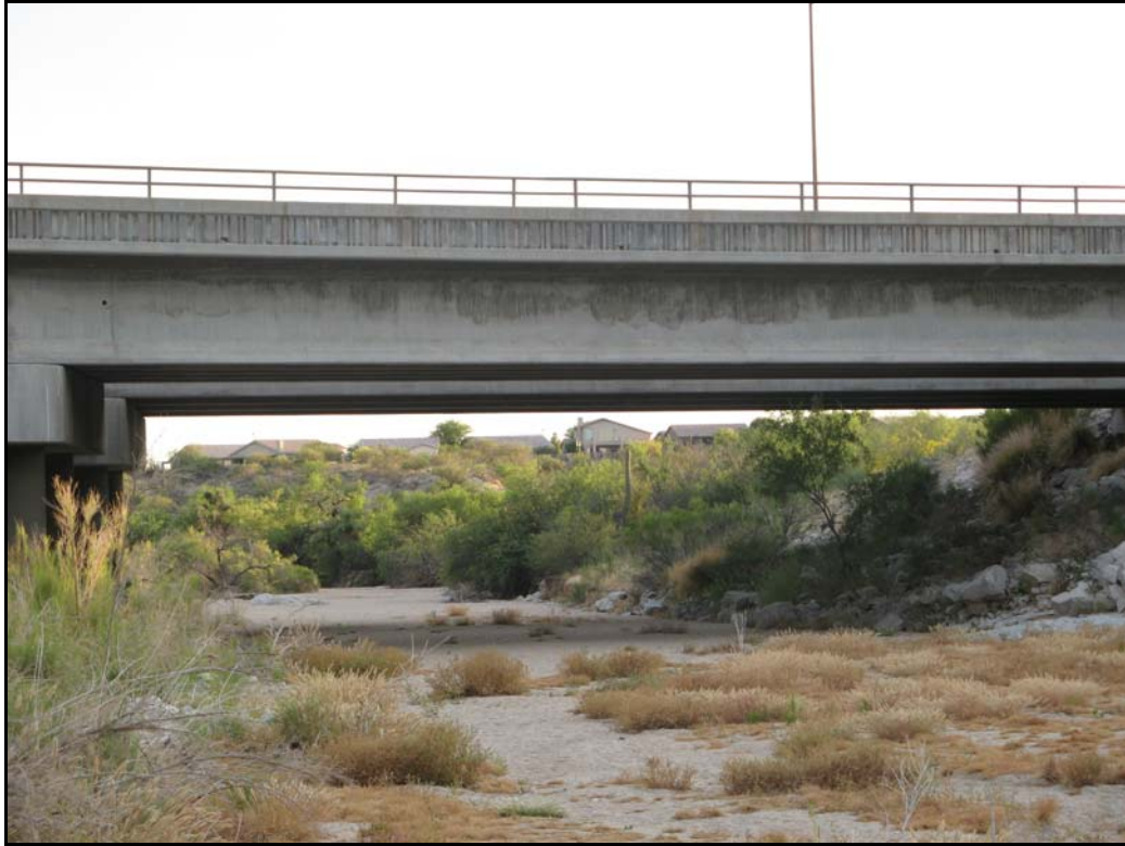
Figure 17: Bridge on RanchoVistoso Blvd over Sausalito Creek (Waypoint 10).
